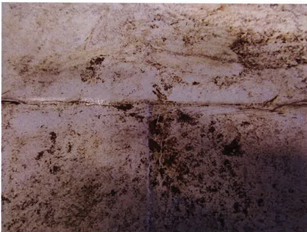
Figure 2: Membrane surface with T-joint
