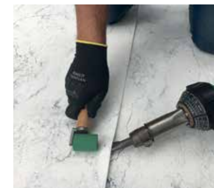
1 st Welding on the inside of the overlap
