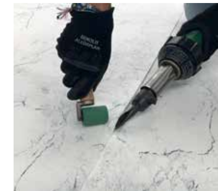
2 nd Welding on the outside of the overlap
