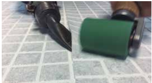
Overlap welded seams
