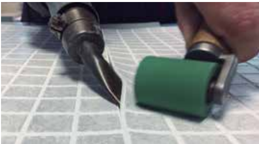
Butt welded seams
