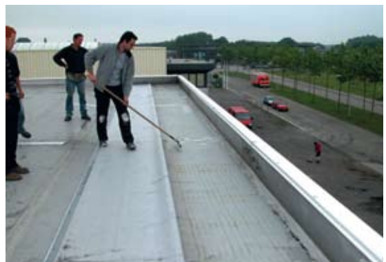
Pict. 2: The glue is dispersed evenly over the surface using a squeegee
