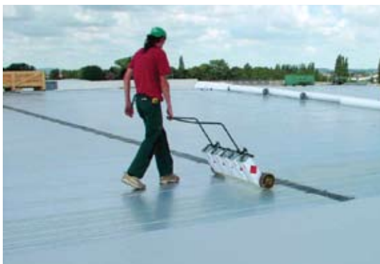
Pict. 1: Application of the polyurethane glue by means of an applicator
