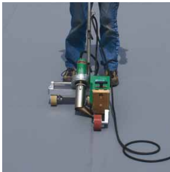
Using a hot-air welding machine
